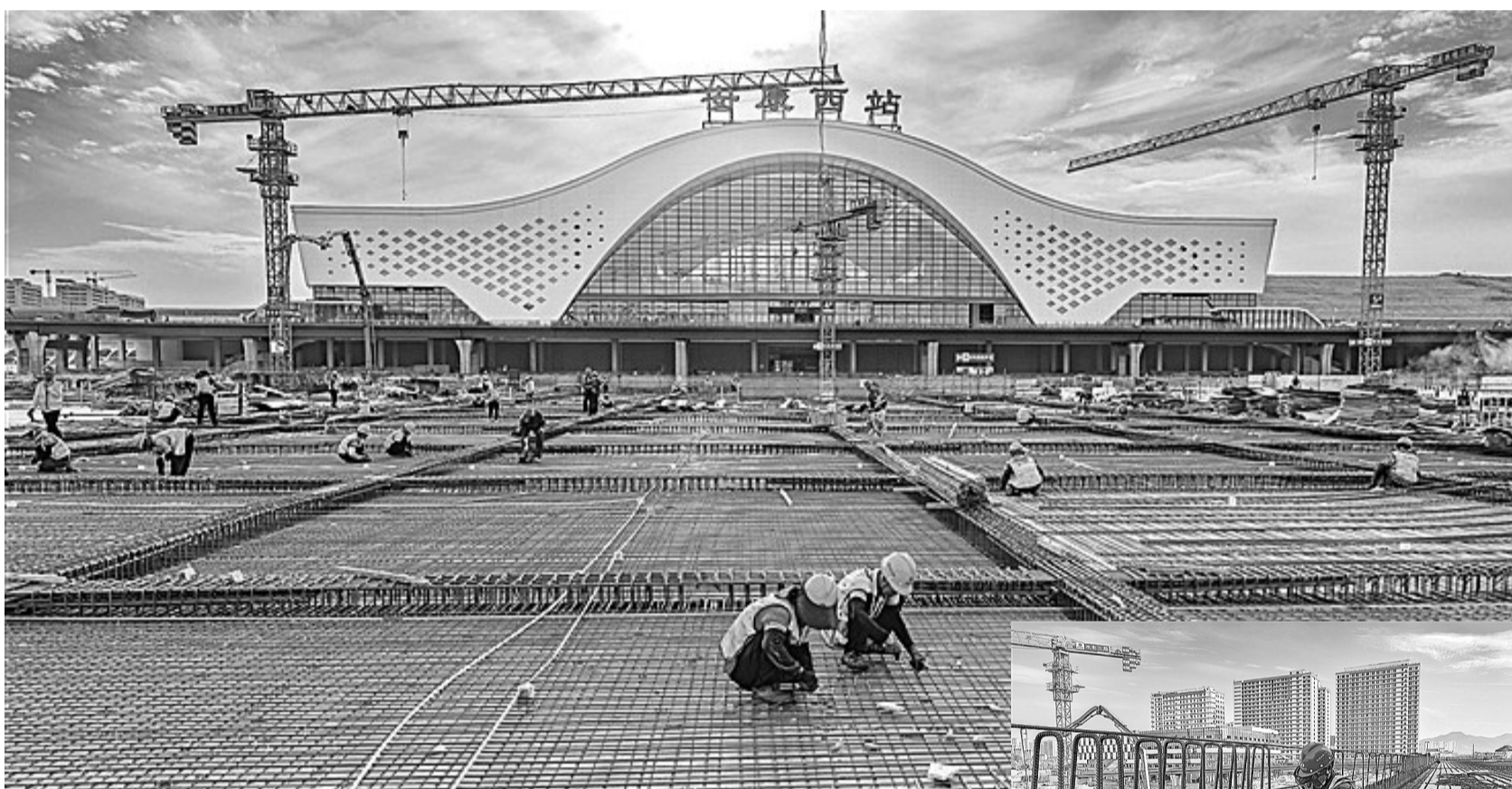
▲工人捆绑钢筋龙骨 ▶工人正焊接高架桥护栏钢筋龙骨
